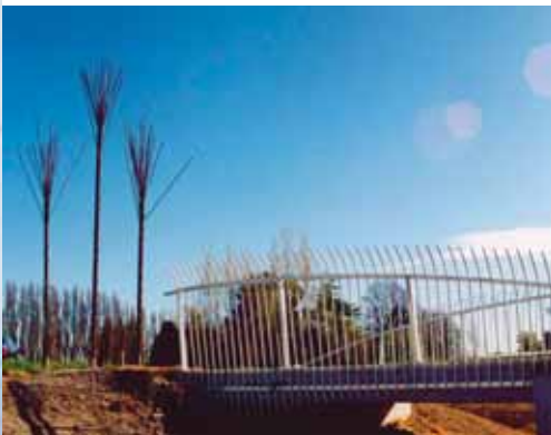
Bridge and artwork, upper Styx River near Crofton Rd
