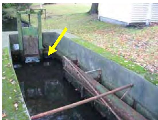
Figure 18. Looking downstream at the old weir at the end of Blakes Road. The centre sluice-gate is open (arrowed).
