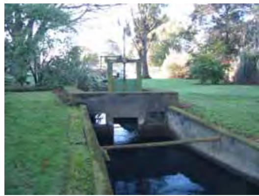
Figure 14. Sluice gate on the middle reaches of the Kaputone Stream.
