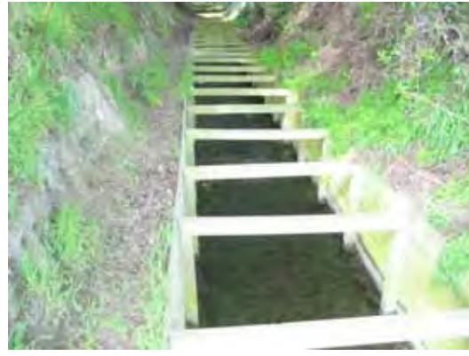
Figure 9. The boxed drain which feeds the excavated ponds in the Styx Mill Conservation Reserve. The drain gravels were used for trout redd excavation.
