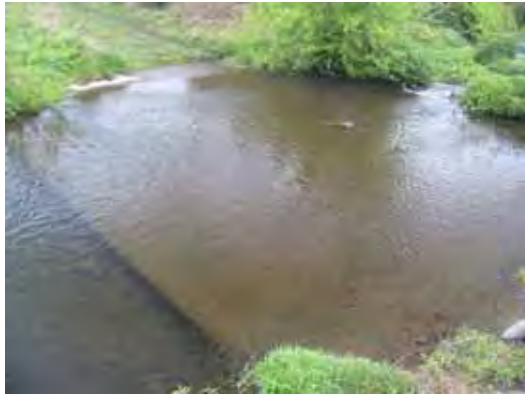
Figure 11. Concrete ford across lake outlet. Water depth was c.a. 7 cm.
