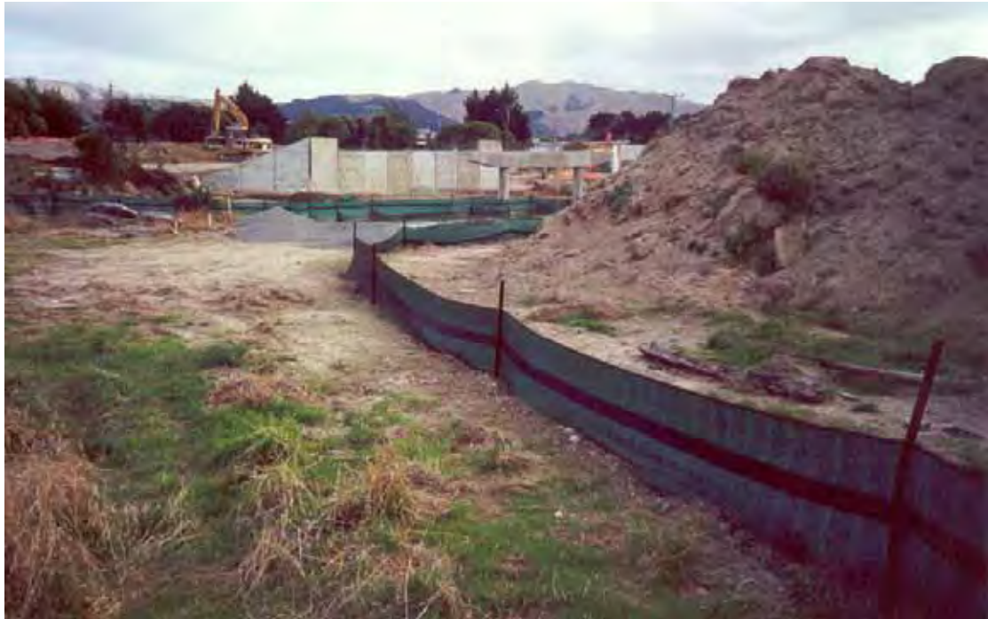
Screening of soil piles to prevent silt runoff during rain events.
