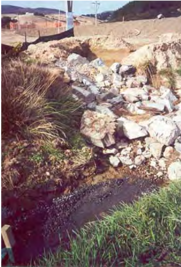
Gravel and screen filter trap to reduce silt from pump water.
