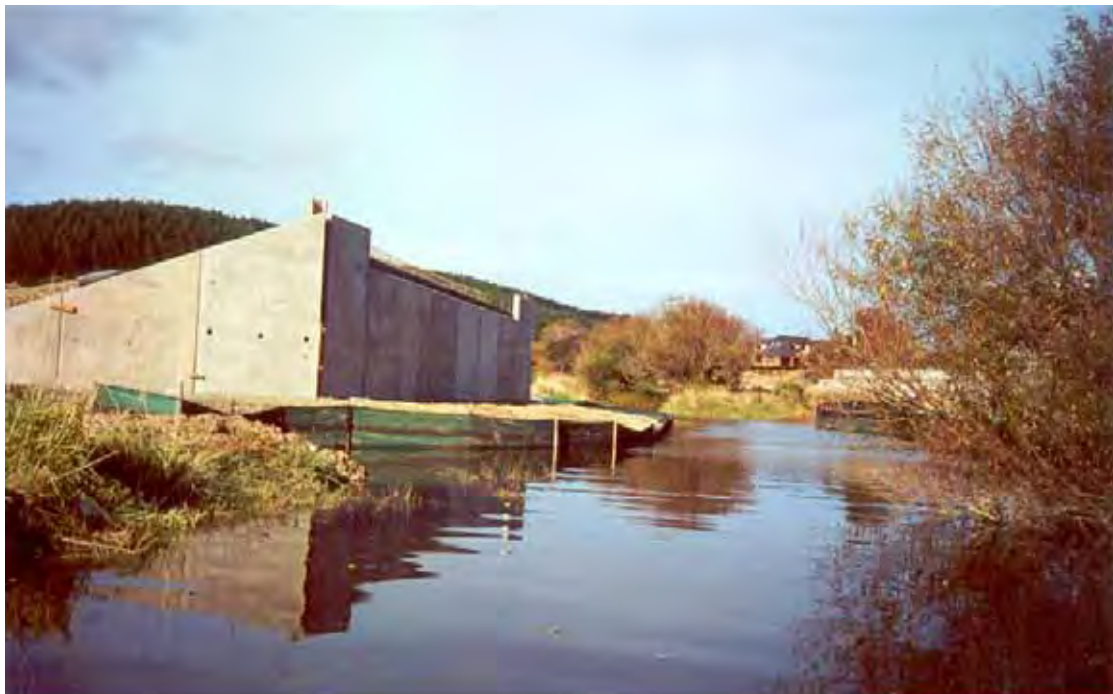
Screening of bridge ramparts to prevent spoil entering the river.
