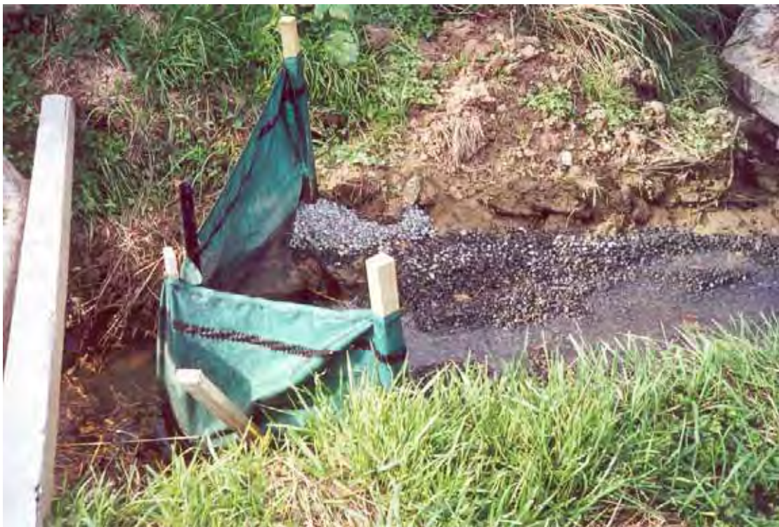
Detail of pump water filter utilising crushed gravel and filter cloth.
