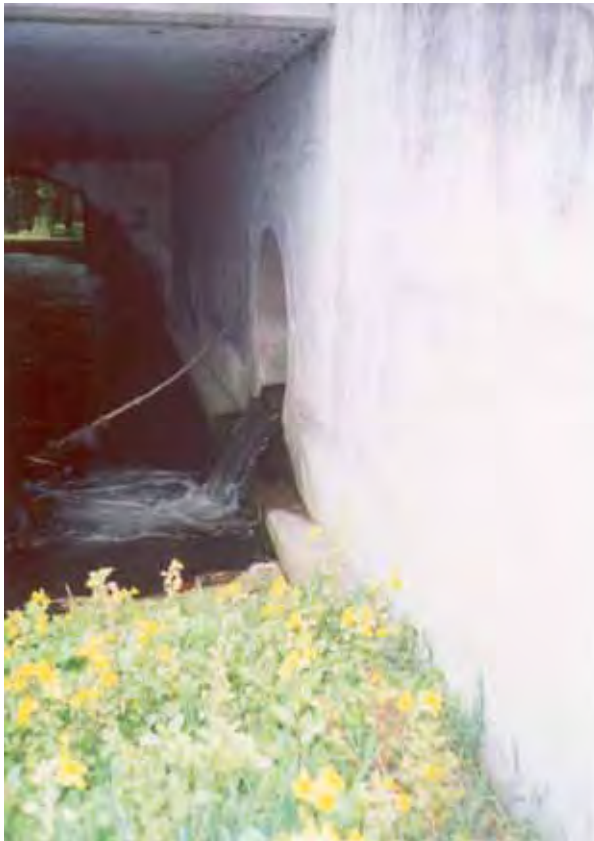
Figure 4. Outfall of the Regents Park culvert into the Styx River. Note the damp spray zone which may allow partial upstream access for eels into the culvert.
